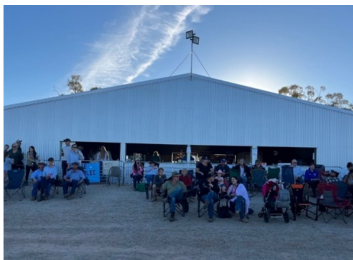
The newly extended and upgraded Balranald Community Hall, which is part of the Homebush Recreation Reserve in the Riverina area of western NSW, was funded by the Crown Reserves Improvement Fund
