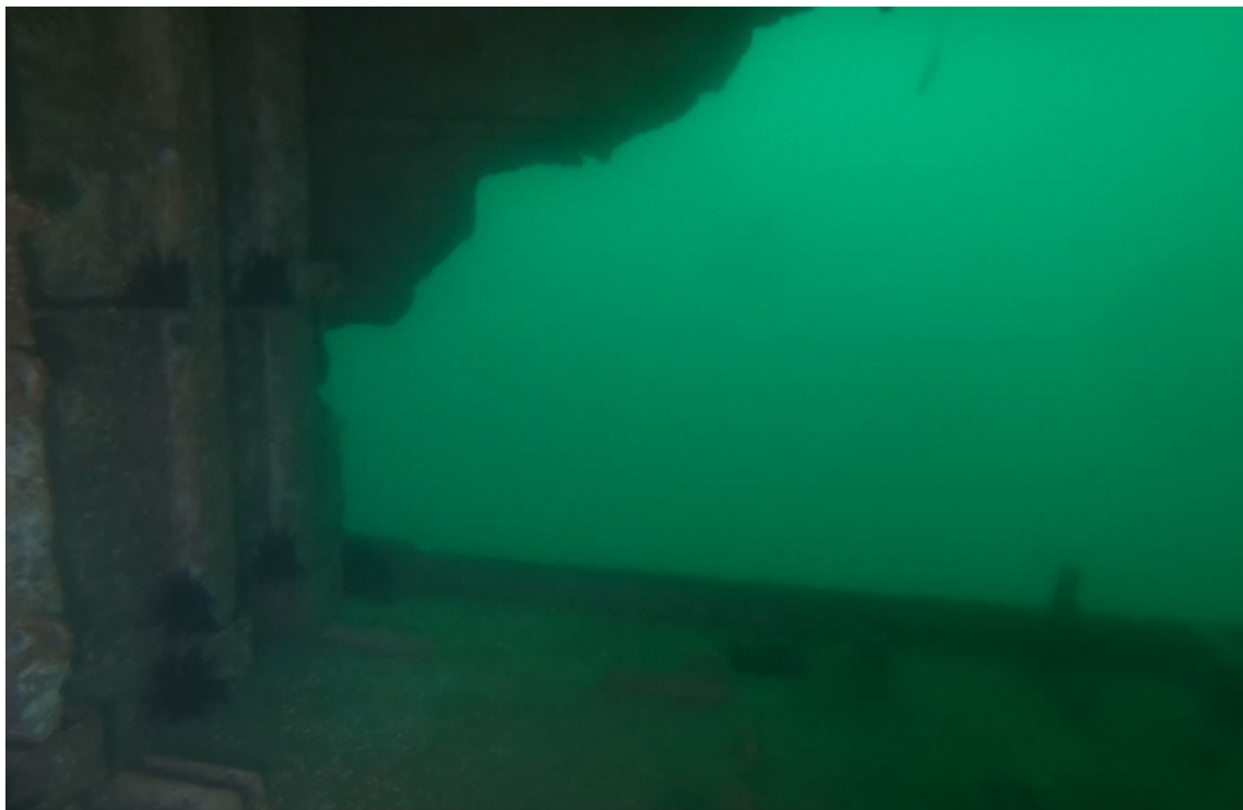
Figure 15: Typical missing outer wall on 01 deck. The aluminum panels have "blown out" in many places. However, it has aided light entry into the interior and has not created new dangers.
