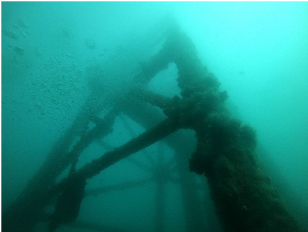
Figure 11: The main mast continues to remain undamaged and all connections are intact.
