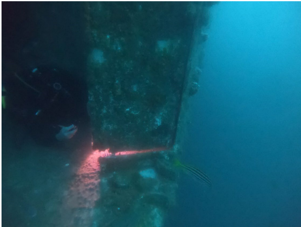
Figure 10: The swinging panel at the starboard walkway through the weather shield.
