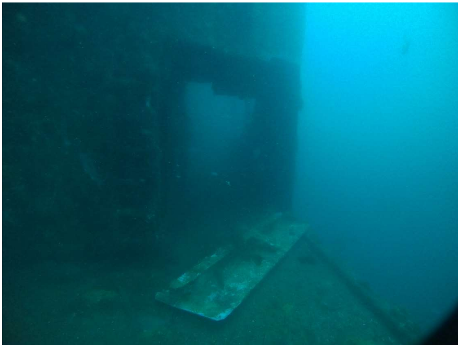
Figure 4: the Weathershield panel after cutting down.
