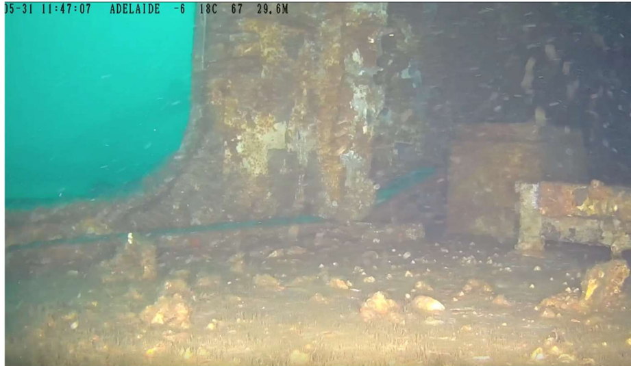
Figure 1: The base of the starboard hanger wall before cutting down.
