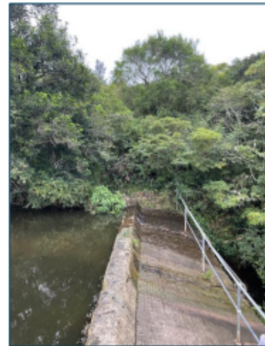
Figure 1. Part of the dam spillway.
