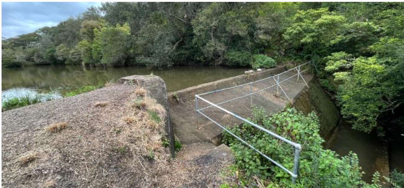
Figure 4.5 Spillway used for access to Lonus Avenue and Whitebridge High School
