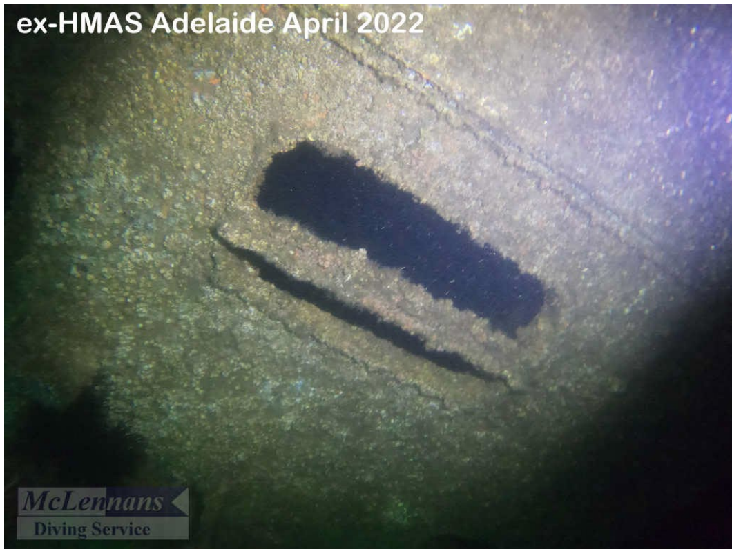
Figure 26: All barred off areas examined had entry bars in place
