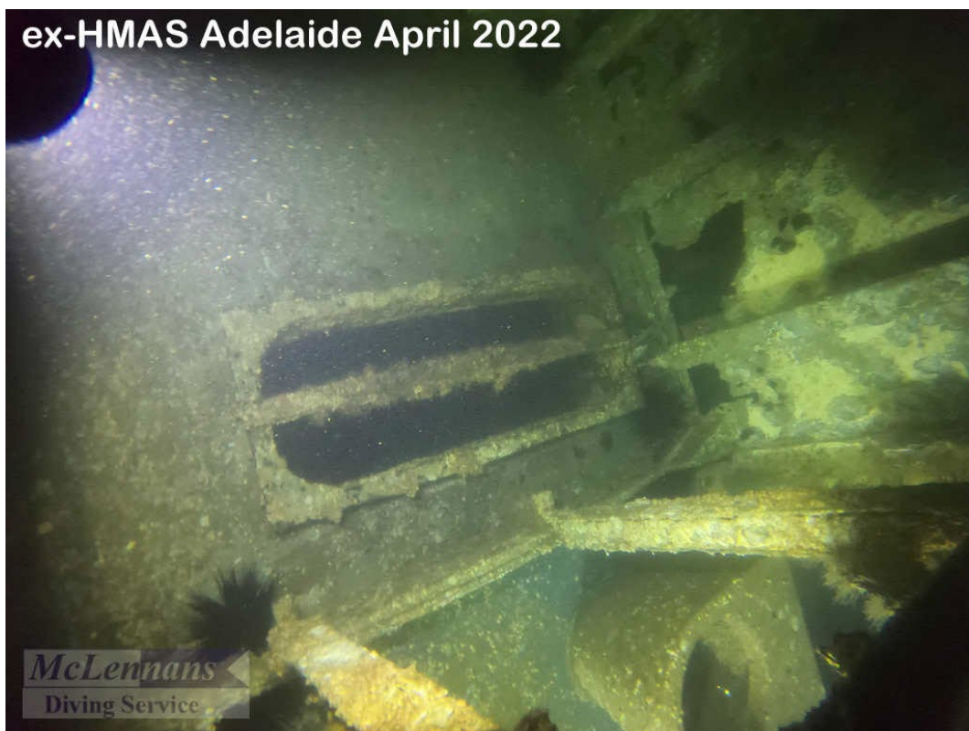
Figure 29: All barred off areas examined had entry bars in place
