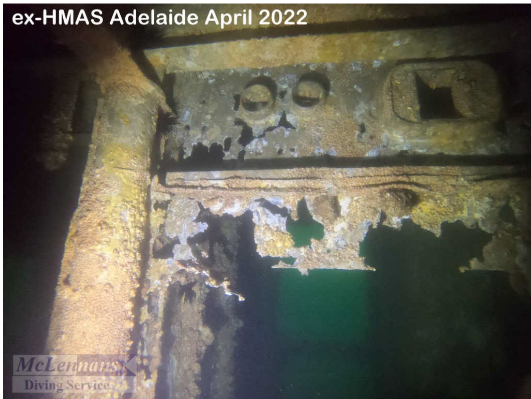
Figure 17: Another view of typical internal wall extreme corrosion. The corrosion is not uniform.
