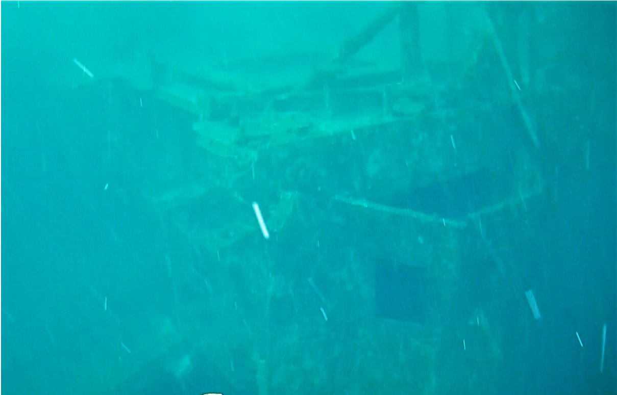
Figure 12: A wide view showing the Flight Deck Observation room and the missing port hanger. The collapsed interior hanger wall is in the bottom left corner. The starboard hanger is to the right.
