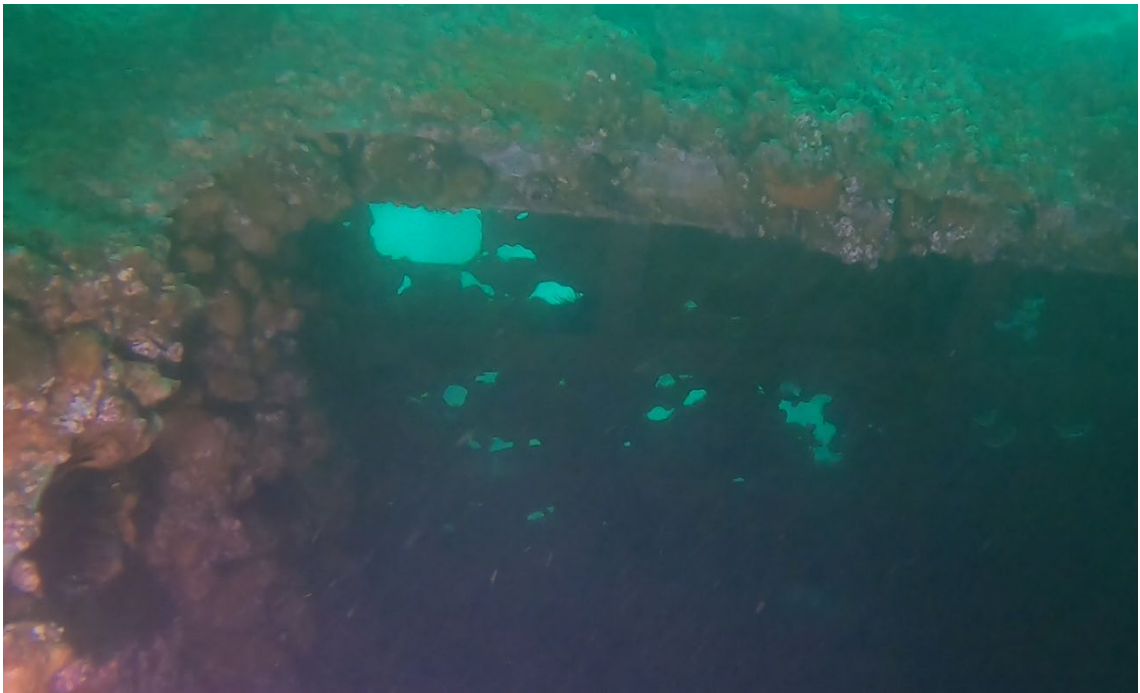
Figure 18: Typical corrosion holes in 02 deck behind the bridge
