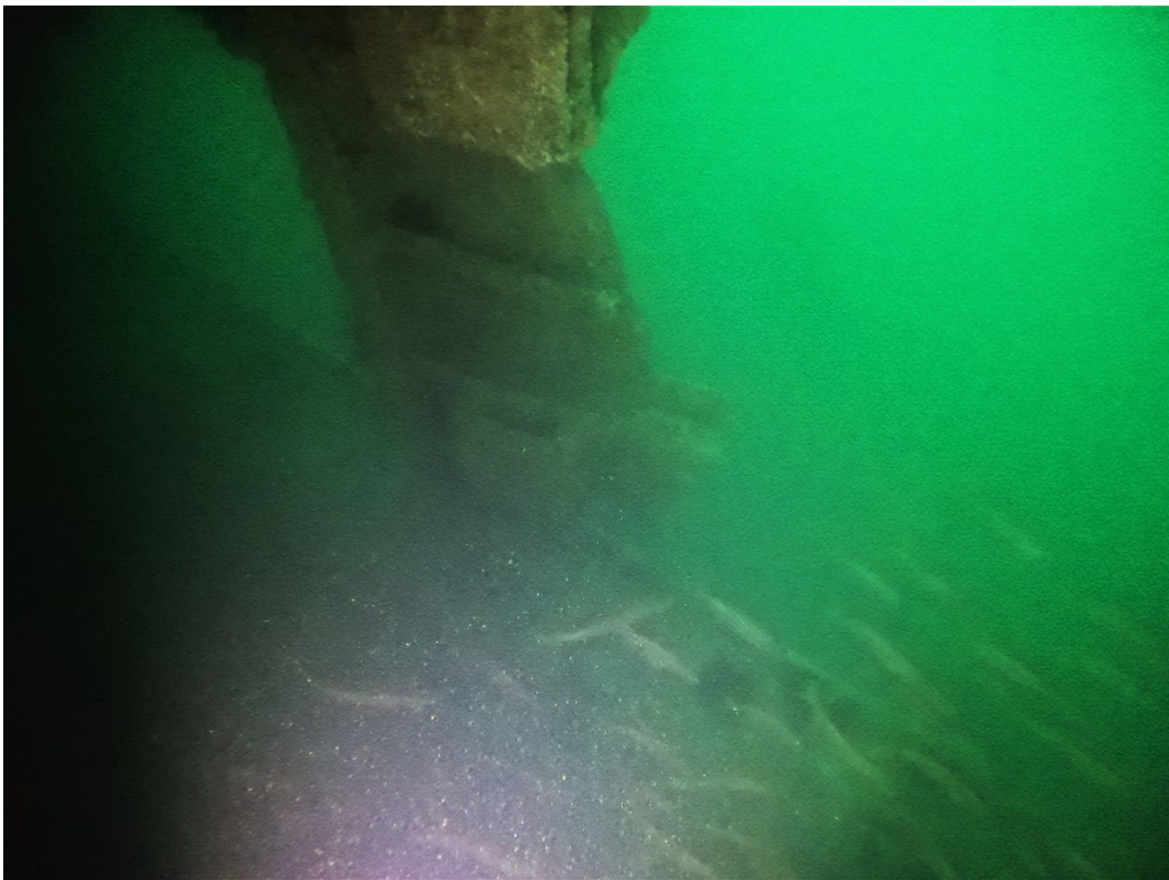
Figure 5: The panel on the starboard wall of the starboard hanger that was removed. There is no support for the starboard hanger
