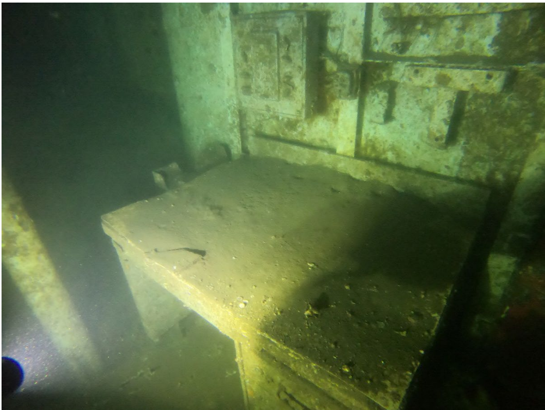
Figure 35: Typical silt deposits in the enclosed compartment on the main deck behind the weather shield. A panel that was opened on the starboard side which should clear this out.
