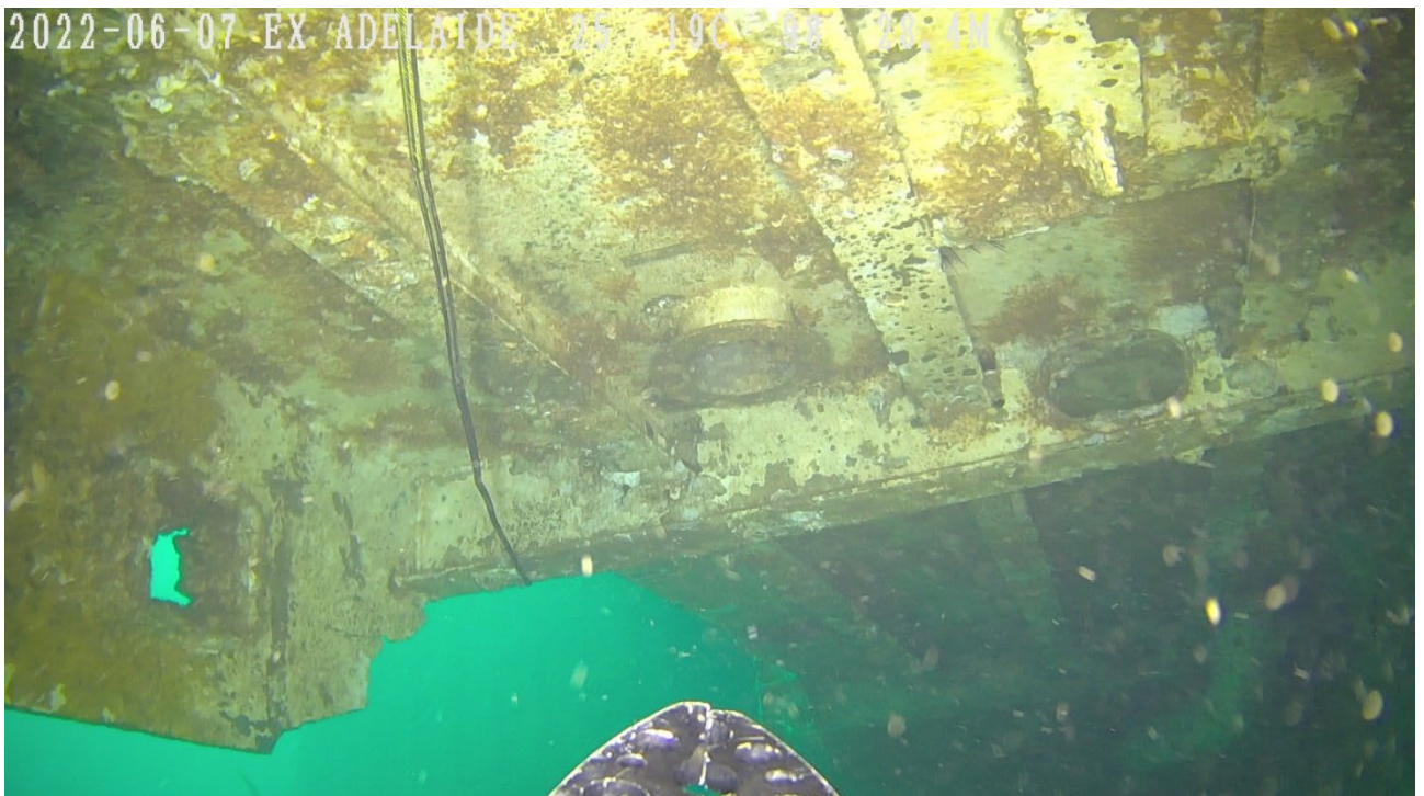
Figure 9: Looking up at the roof of the central companionway. This is the floor of the 01-deck companionway. The interior hanger wall was to the left.
