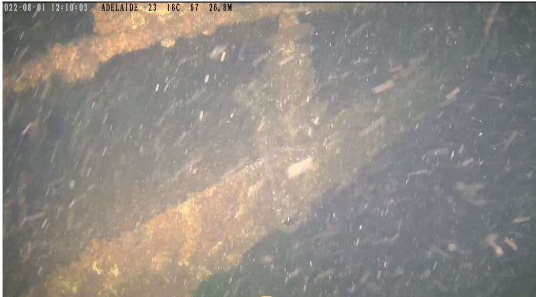
Figure 4: The catwalk in the starboard hanger which is adding strength to the roof.
