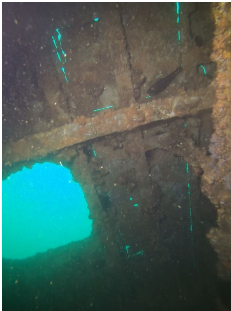
Figure 1: Looking up at the starboard hanger roof. Note the many corrosion holes.
