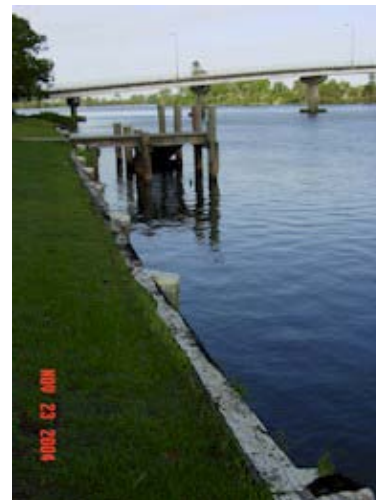
Figure 12 Riverbank reserve access showing sudden, steep drop into river.
