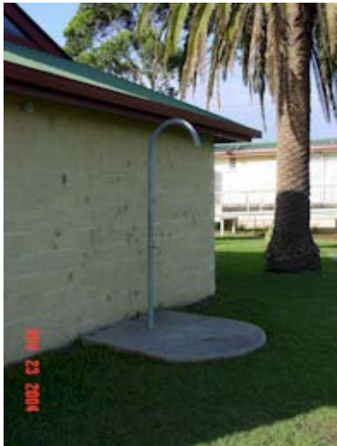
Figure 6 External Amenity Block Shower.
