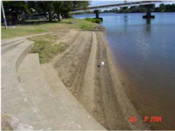
Figure 14 Constructed Beach. Tyre protection located at far end of beach.
