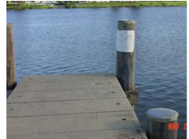
Figure 9 Jetty Safety Sign requiring replacement (Blank sign).
