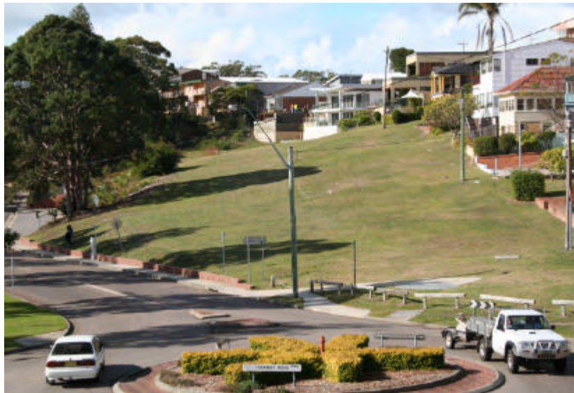
Photograph 5.3 Embankment near Teramby Street roundabout
