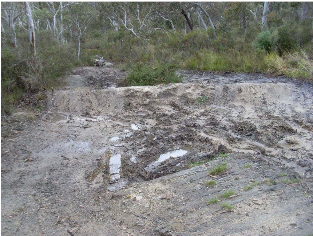
Plate 14: Track proposed to be closed due to erosion and proximity to hanging swamp
