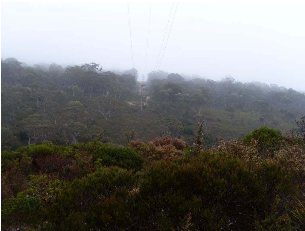
Plate 7: Same location as Plate 5 facing east along the electricity easement
