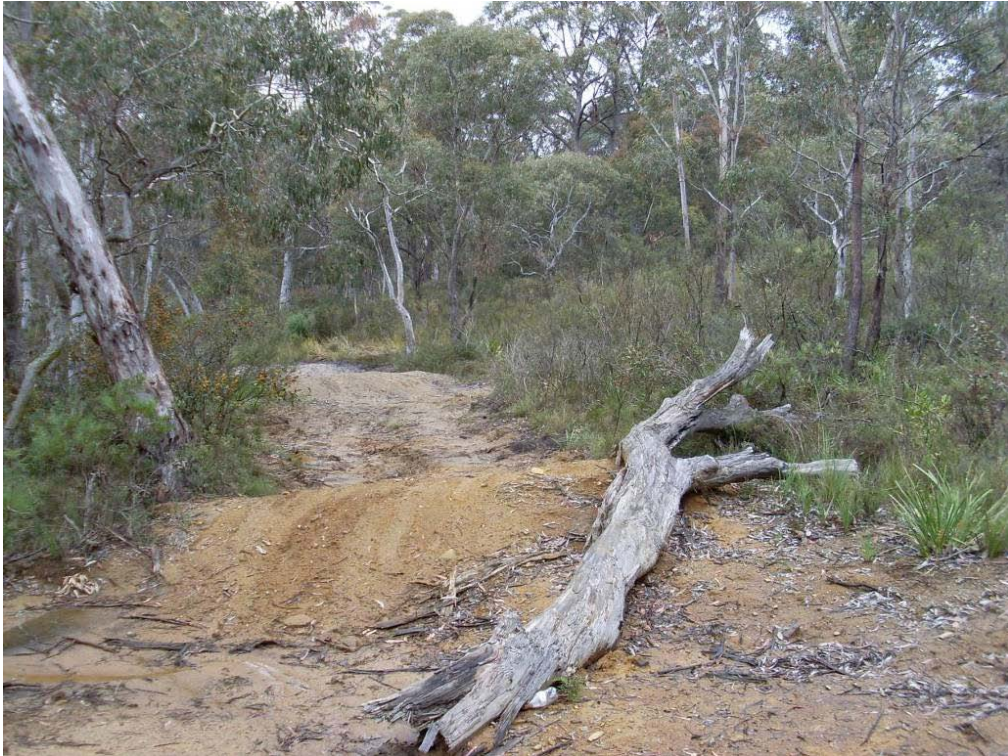
Plate 13: Access track from the railway corridor to the lower dam
