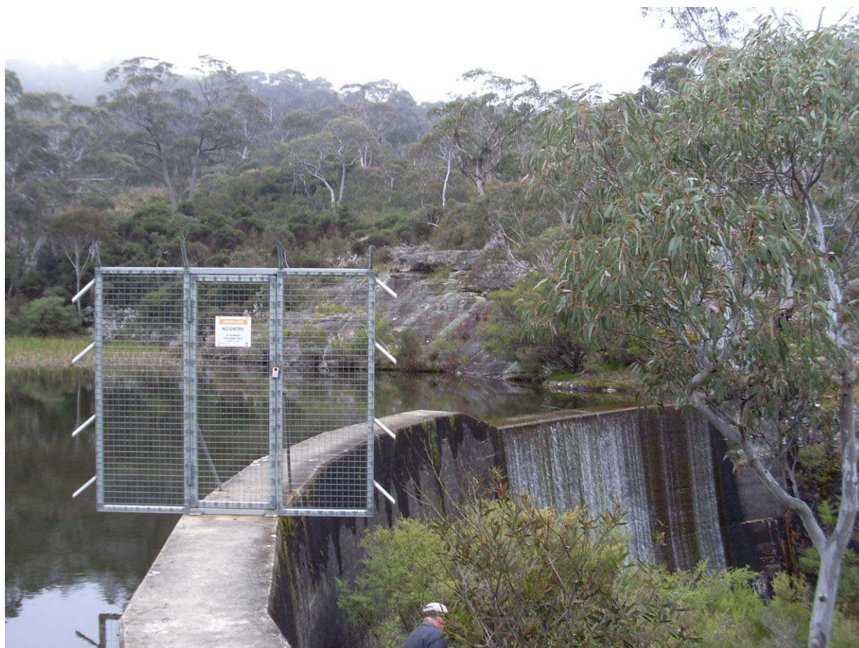
Plate 3: Gate installed to prevent people walking across the dam wall of the lower dam.
