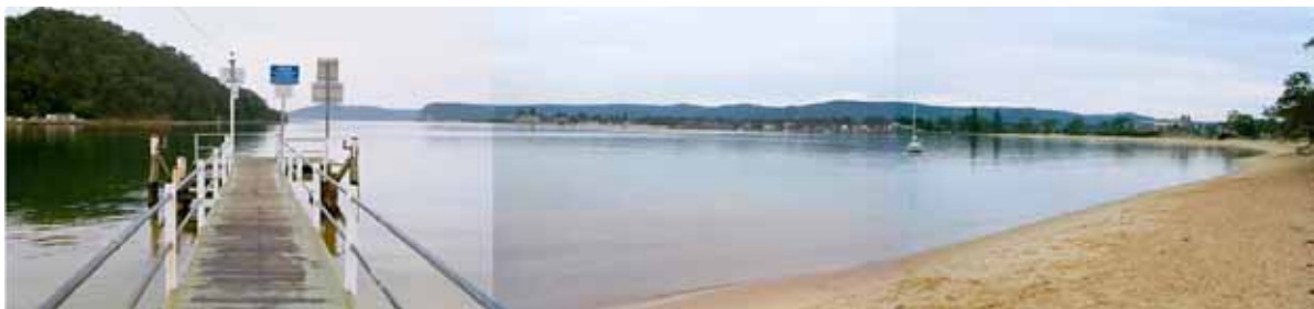
Figure 36 - Existing Ferry wharf at Ferry Road looking south-west
