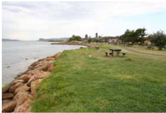
Figure 29 - Rock wall looking south
