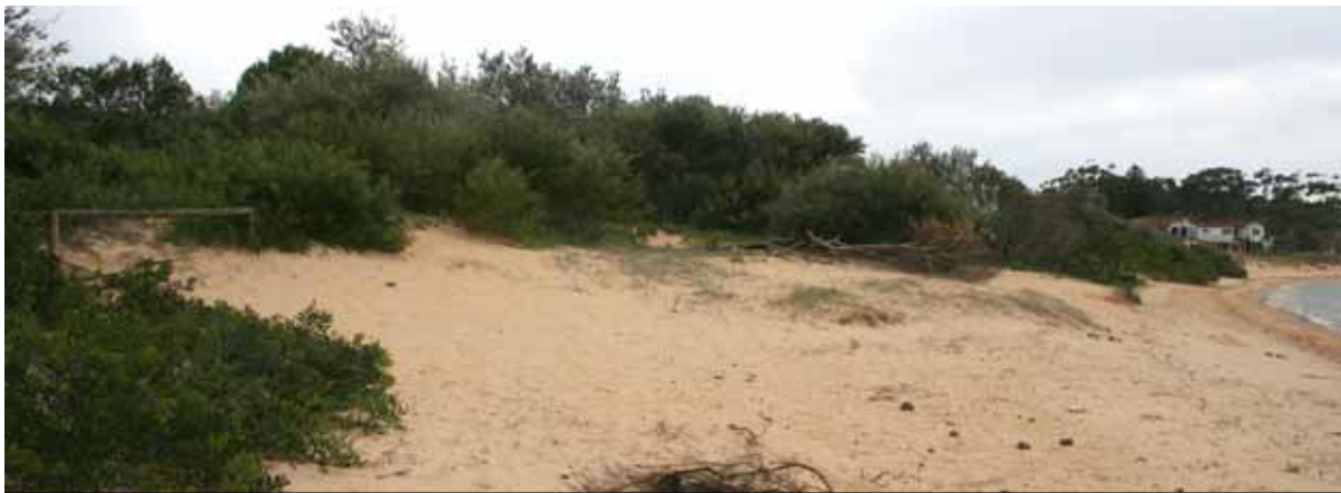
Figure 32 - Dune stabilisation work near Memorial Avenue
