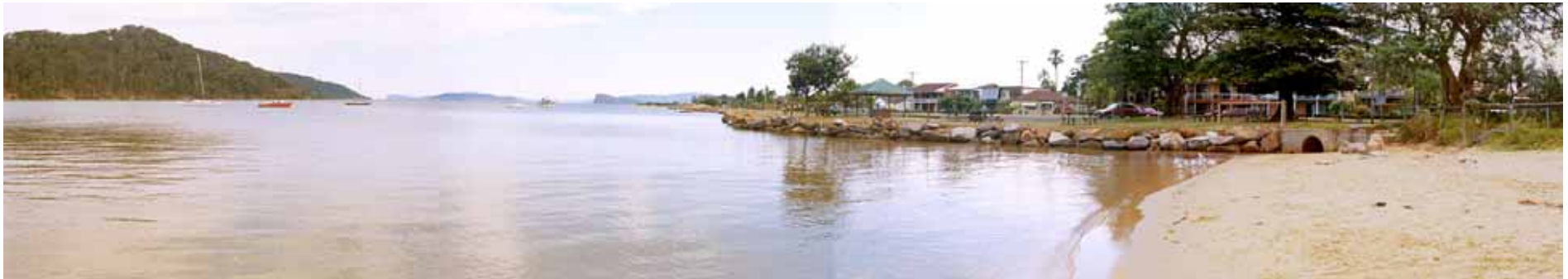
Figure 37 - Broken Bay View with the rock revetment, foreshore park and Beach Street stormwater outlet to the right
