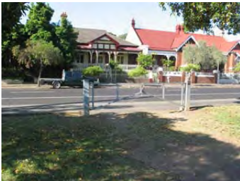
Vehicular access gate
