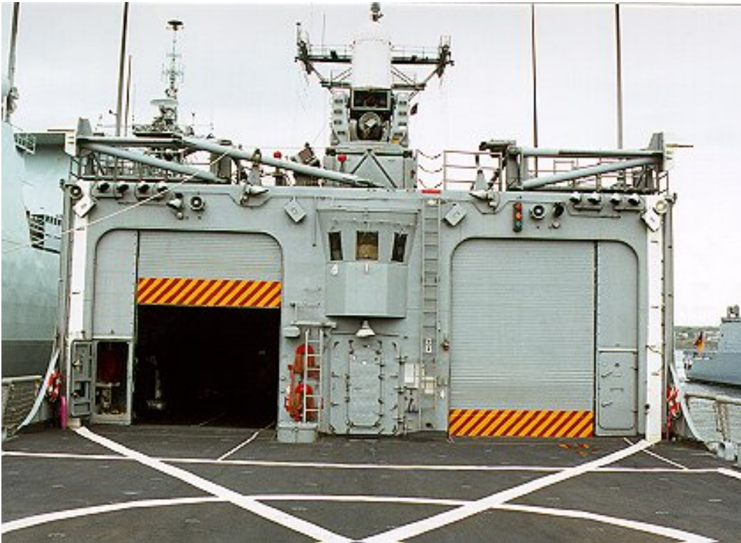
A view of an FFG flight deck with the observation point visible and the guy pole for the davits attached above it
