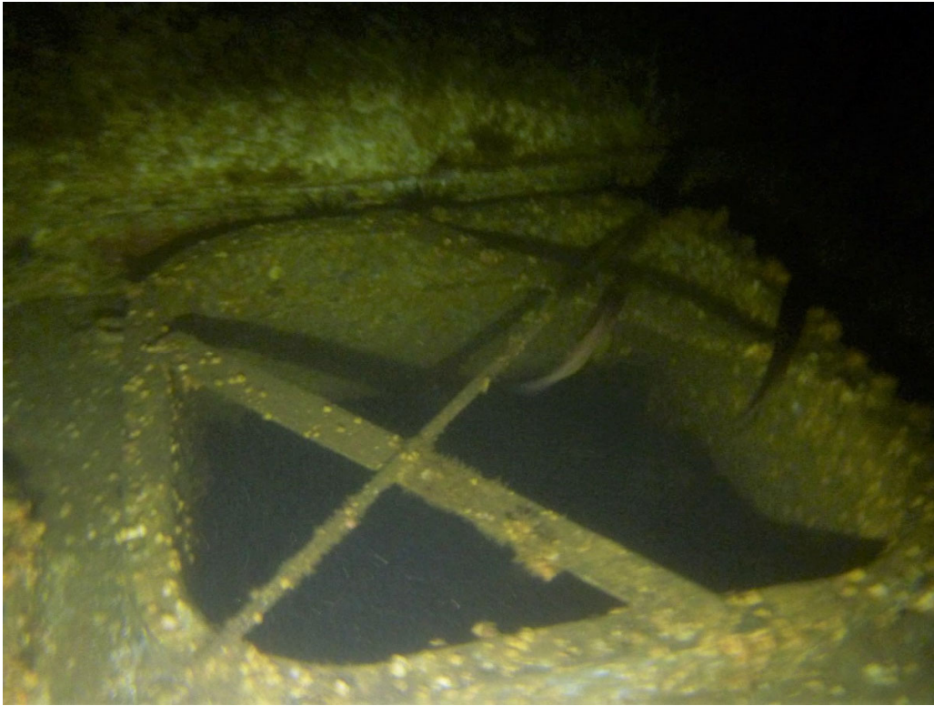
Figure 10: Passageway 1-212-0-L Frame 247 - All bars intact
