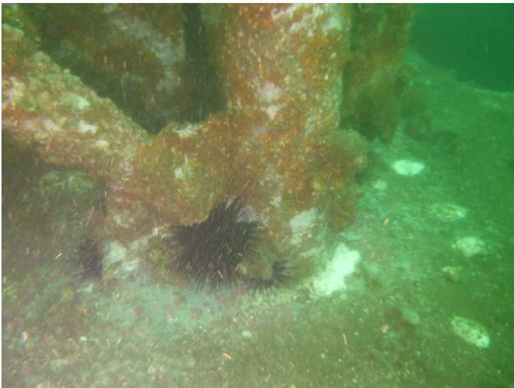
Figure 16: A similar view of another leg of the main mast
