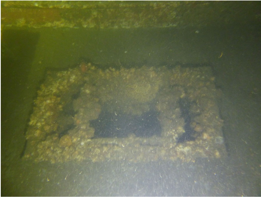
Figure 8: 400Hz Freq Changer Room Frame 262 - Bars in place
