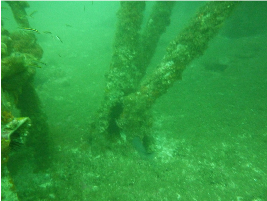
Figure 15: A view of one of the main mast legs showing a sound connection to the superstructure.
