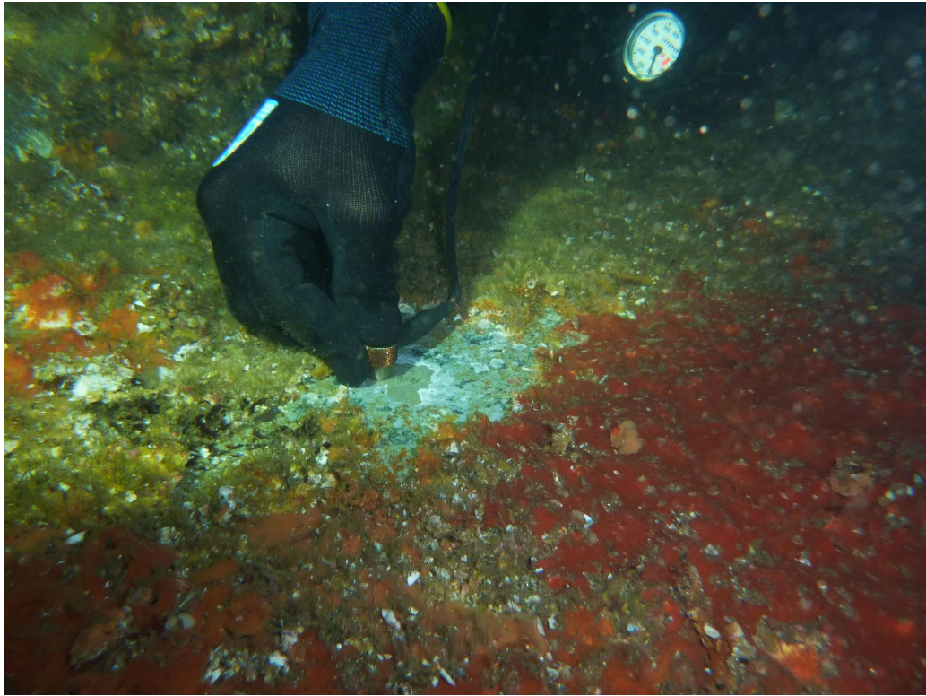
Figure 3: Close up of thickness testing location on Starboard side amidships. Note the grey hull paint still intact
