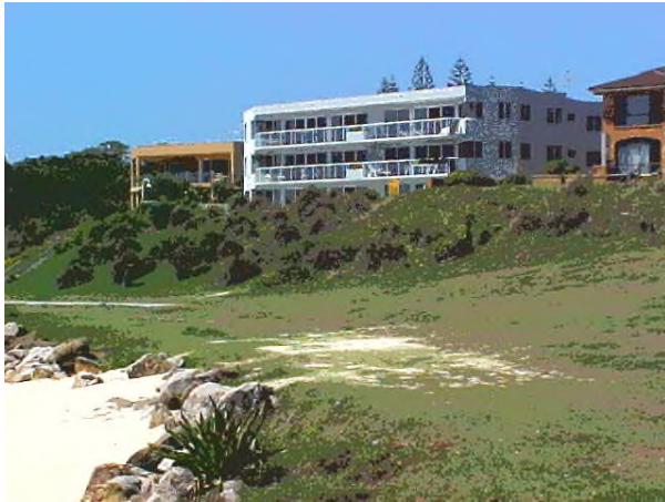
Holiday units “Lees Court” near Saltwater Creek entrance
