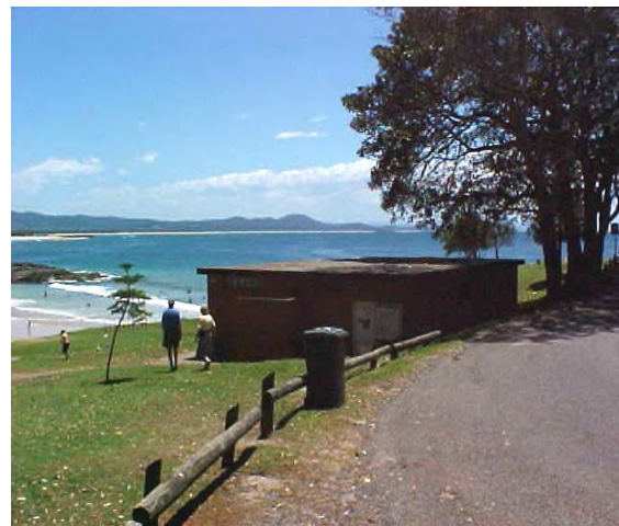
Main amenity block along access road
