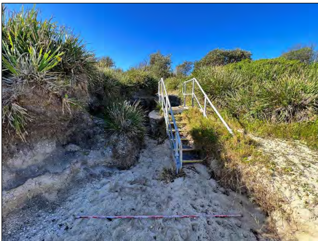
Plate 9: Eroded walking track and staircase.
